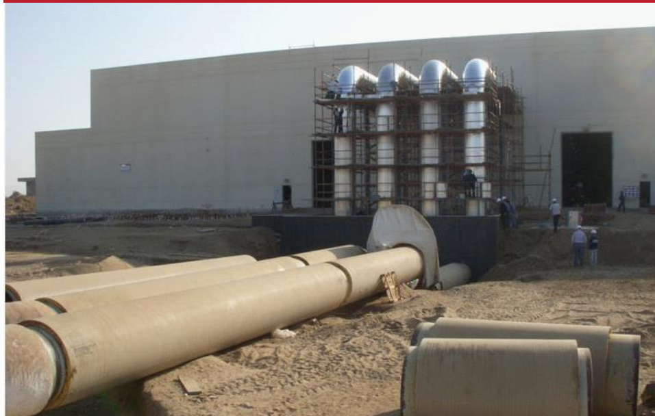
MECHANICAL CONNECTIONS TO CENTRAL COOLING PLANT
