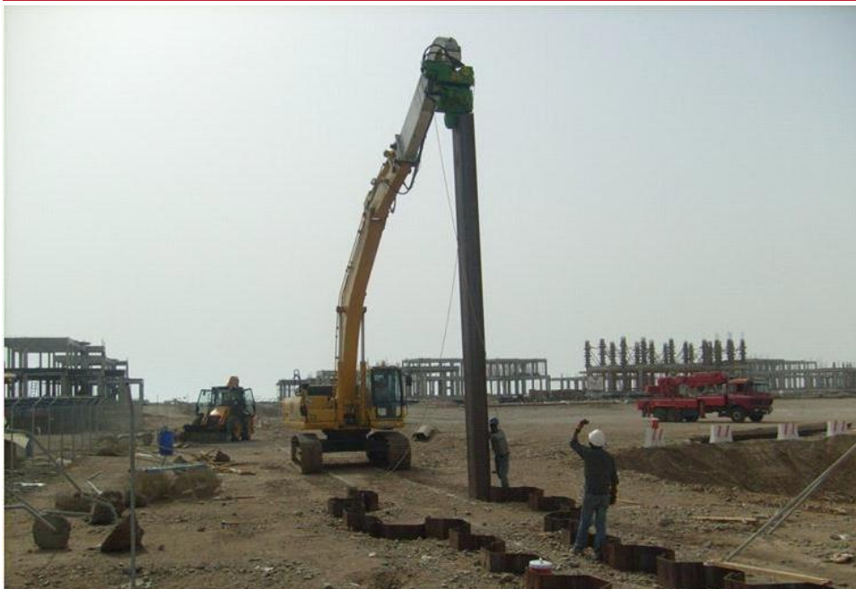
SHEET PILING FOR DEEP EXCAVATION
