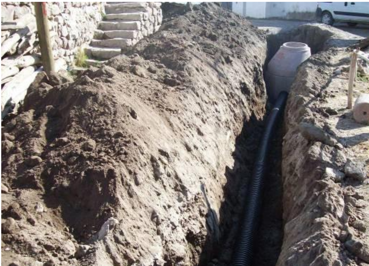
Ø200 HDPE CORRUGATED PIPELINE
